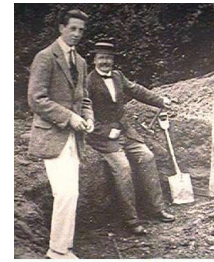
Hinton (left) and Dawson (right) at the site.
